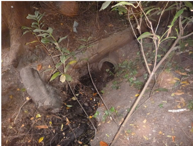
Figure 2. Photo showing stream outlet from culvert.
